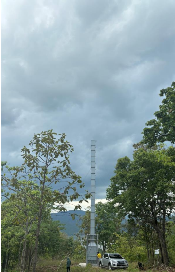
Before of the operation 02.00 p.m.
